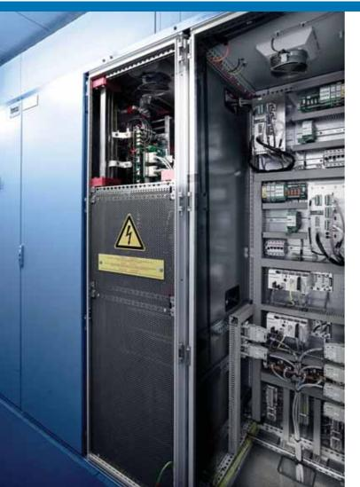
The Bentec VARIABLE FREQUENCY DRIVE is a state-of-the-art converter technology developed for the special operational requirements on drilling units. Because it has been self-developed by Bentec, the VARIABLE FREQUENCY DRIVE provides an absolutely reliable system for drilling applications.
